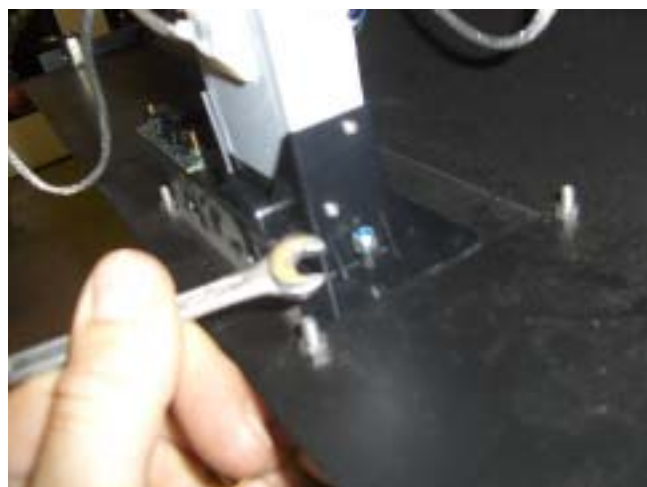
Figure 4. Securing New SmartCard Reader In Place
