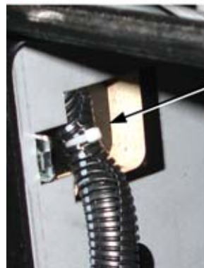
Through hole into Coin Vault.
